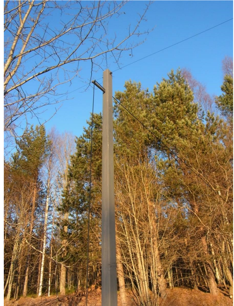
Top of the front pole
