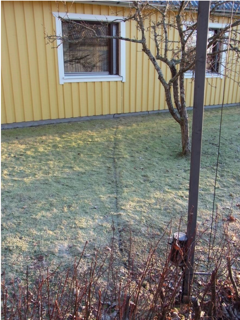
Coax RG-213 just a few centimeters under the lawn leading to the receiver
